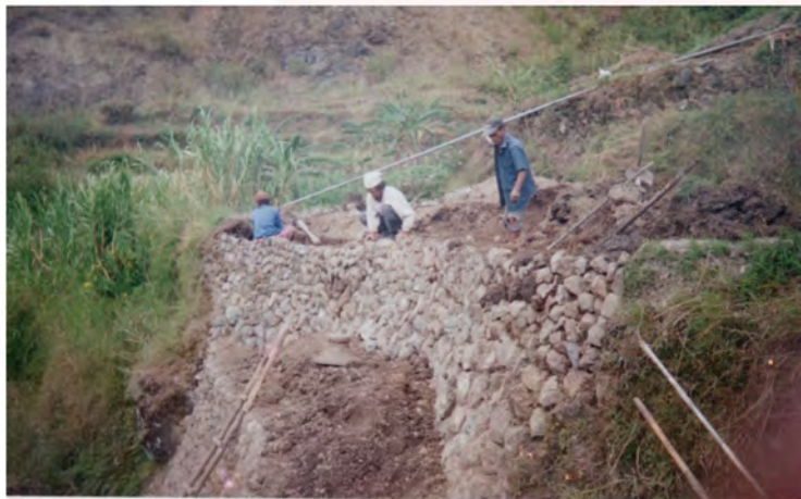
Local construction of Stone Walls using traditional Indigenous practices © W. Alangui
